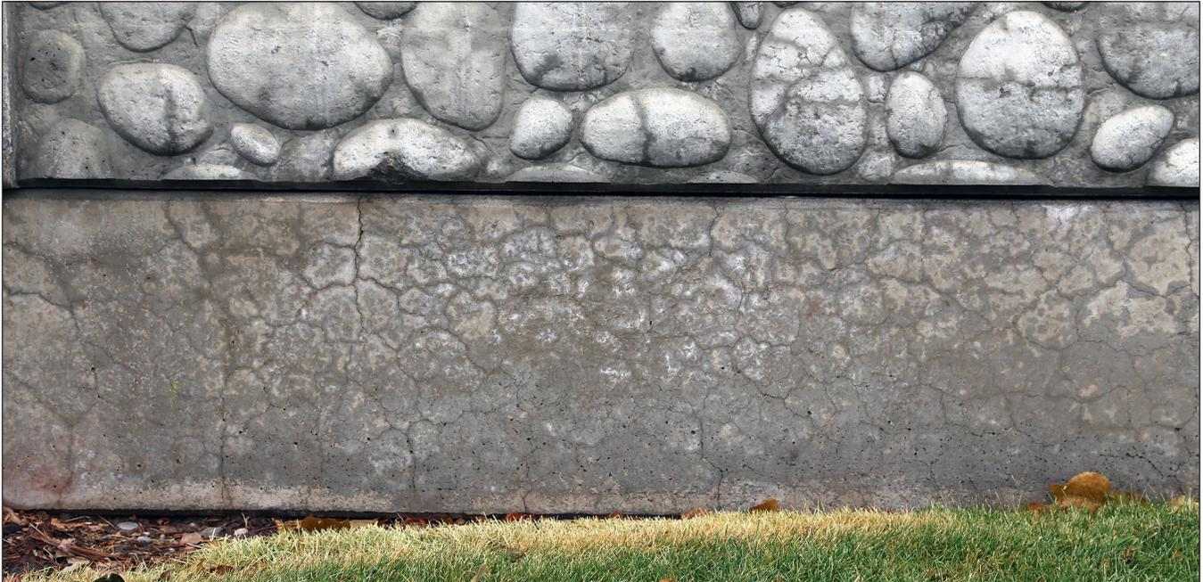
hard facts are these: ASR-affected concrete is flawed at the molecular level and will not reach its engineered lifespan.
