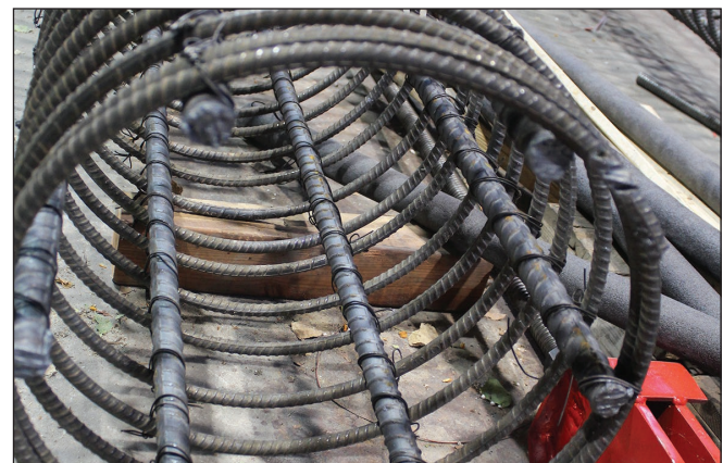
Rebar cage for bridge support column
